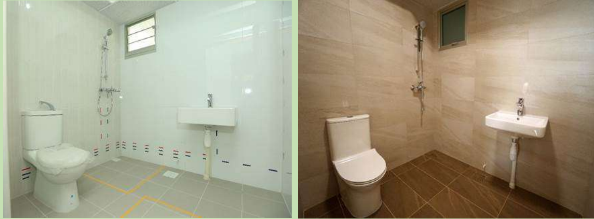
Existing WCs and wired-glass louvered vent windows (left), will be replaced with dual-flush low-capacity WCs and top-hung windows (right).
