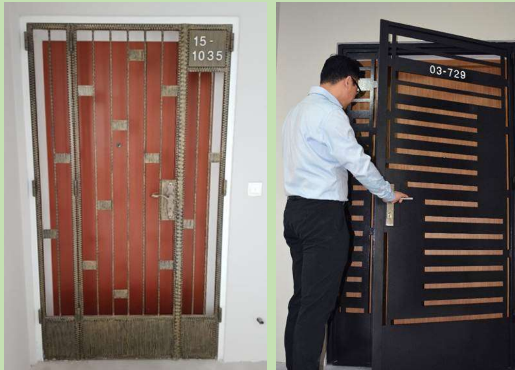
Existing timber veneered doors and wrought iron gates (left) will be replaced by laminated timber doors and steel entrance gates for a more contemporary look (right).
