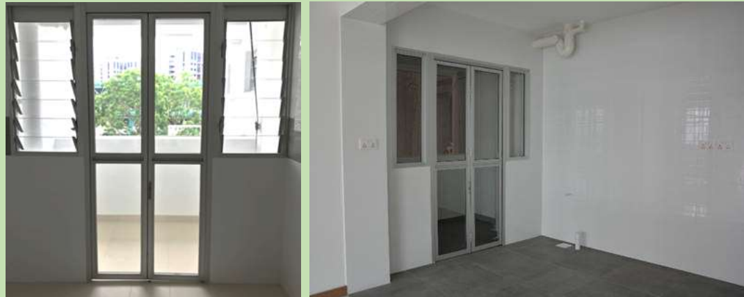
The louvered windows in the door/window ensemble between the kitchen and service yard (left) will be replaced with top-hung windows (right), allowing for more flexibility in the layout of kitchen furniture.
